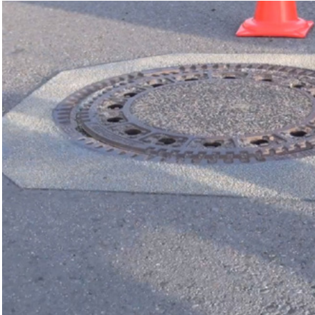
Grouting and masonry mortar
