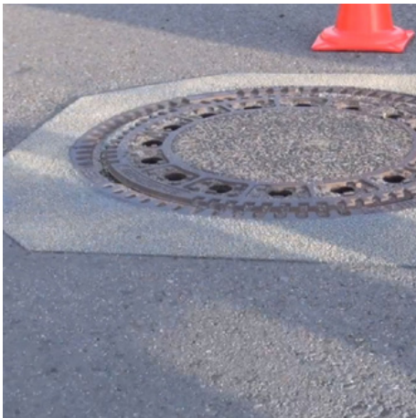
Grouting and masonry mortar
