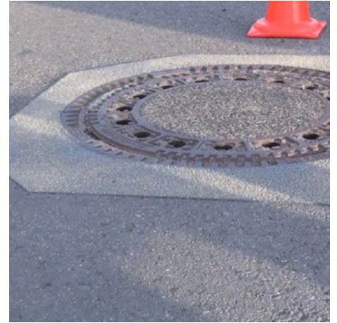
Grouting and masonry mortar
