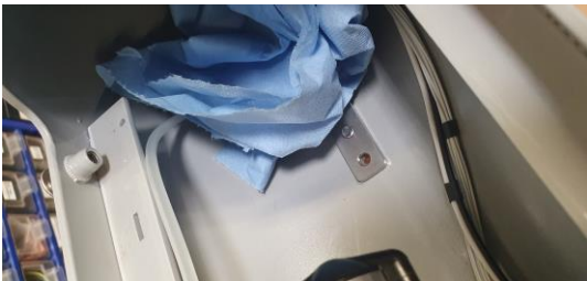
Figure 42 - cleaning of the turbine compartment
