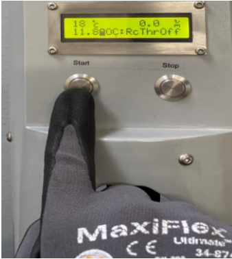
Figure 14 - Step 4: Start-up of the turbine
