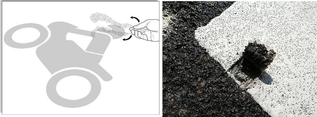
5. The material cools normally within 5-10 minutes. When the material has completely cooled an adhesion test can be performed with a hammer and chisel. Good adhesion is achieved when parts of the asphalt surface has adhered to the back side of the marking (see picture above). To speed up the cooling during hot days sprinkle with some water. Remove surplus/ non-attached glass beads after application is completed.
